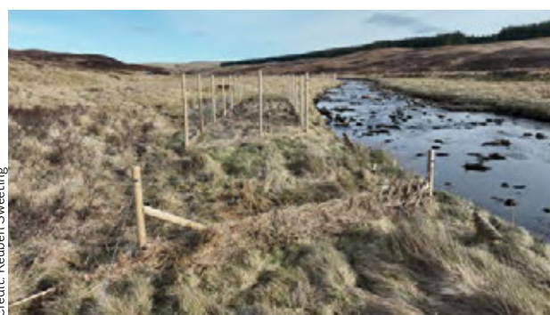
The sacrificial fence is doing its job by protecting the main enclosure and catching debris
