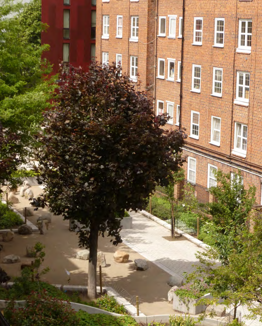
Sustainable Urban Drainage Scheme developed at Percival Triangle in London Islington.
