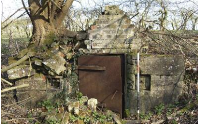
A view of the 'Tar Tank' showing the iron door to the furnace located beneath the tank
