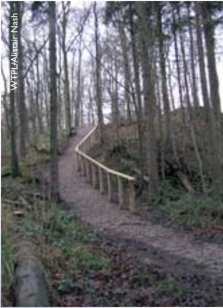
Part of the recent path upgrade in Skipton Woods
