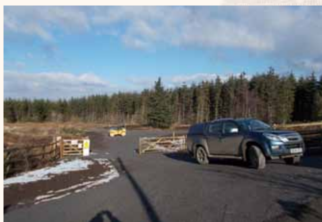
After Mardon down improvements for oversize machinery
